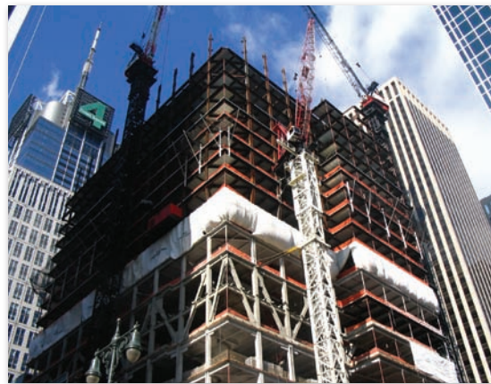
1 Bryant Park under construction, New York City.
